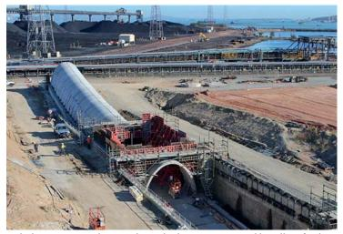
Gladstone Port Authority job Stockpile 22 is a new coal handling facility being built by Hutchies which includes a 165 metre tunnel.
